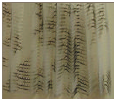
Burnt polymer pleat support mesh from arcing
